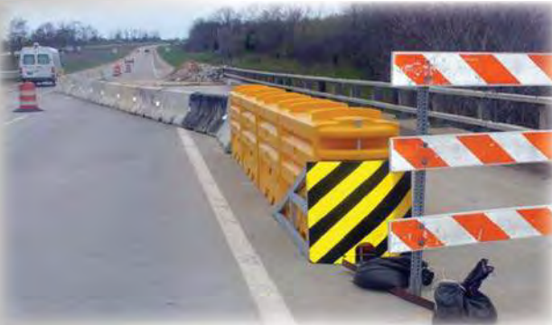
SLED™ TL-3 in use on a Missouri Highway
